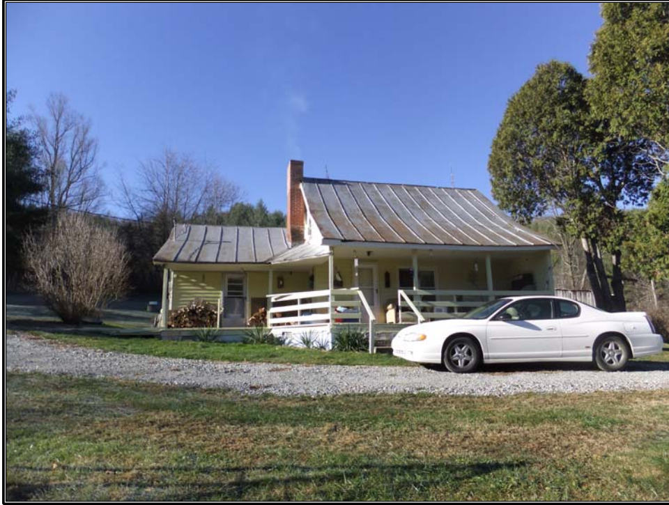
Figure 6. James Weaver House (AL 75): Southwesterly view of residence.
