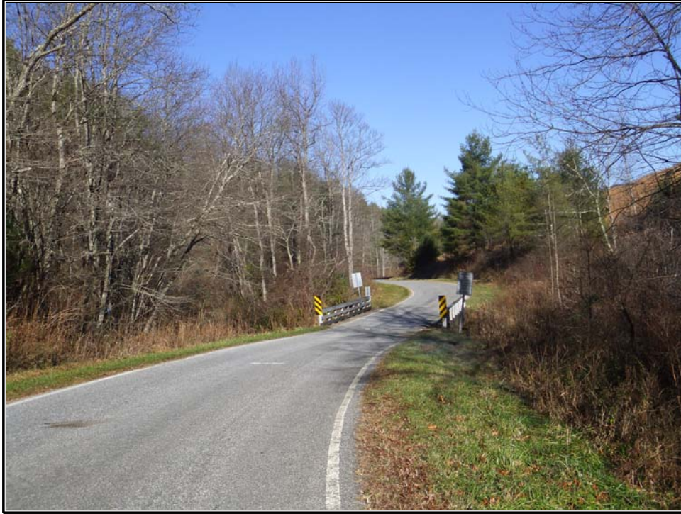
Figure 5. Northwesterly view of Bridge No. 46 over Prather's Creek.
