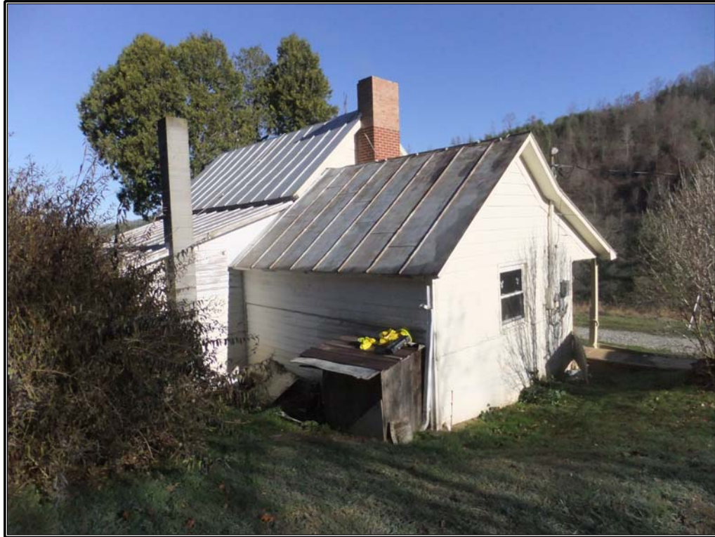
Figure 9. James Weaver House (AL 75): Northerly view of side and rear additions.
