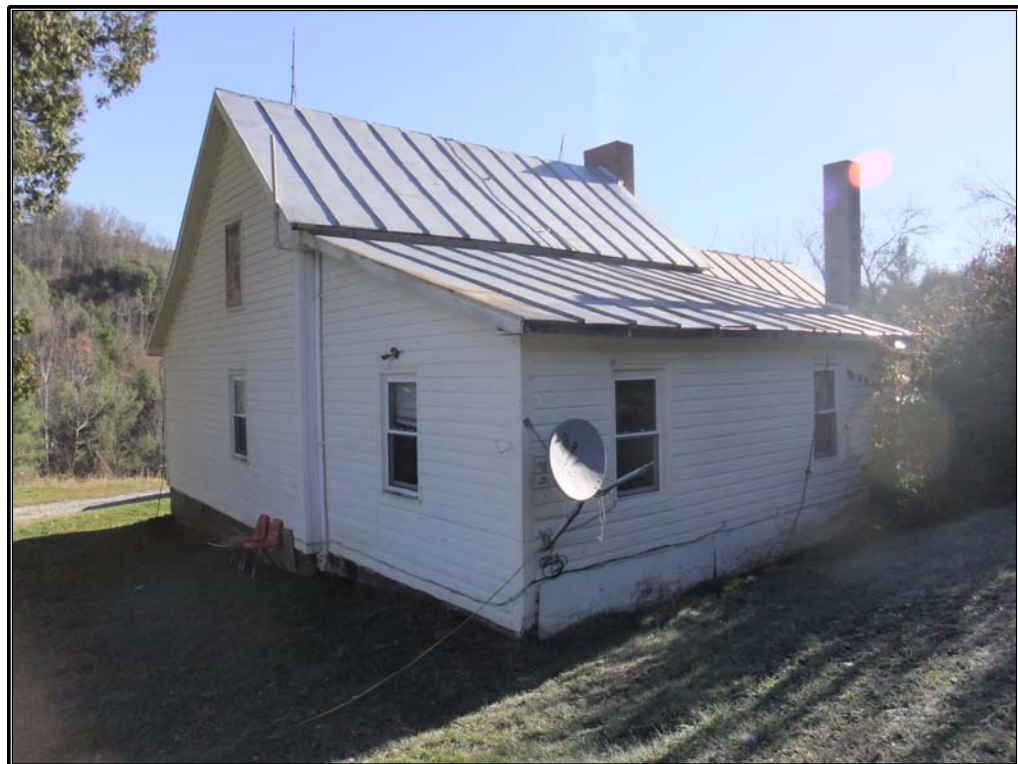
Figure 10. James Weaver House (AL 75): Northeasterly view of rear addition.
